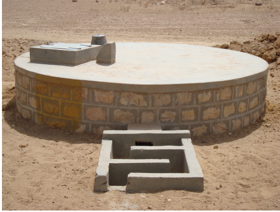
Figure 5: A traditional rainwater harvesting system in Thar desert of Rajasthan, India. (Public Domain, Wikipedia)
